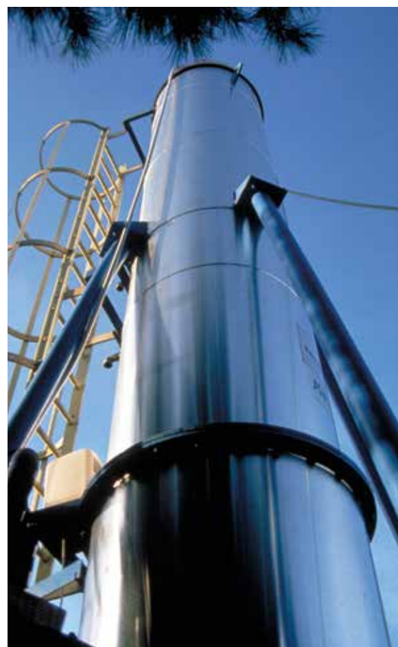
Pollution control, fluidised bed anaerobic digester. INRA-Degremont collaboration © INRAE, R. Moletta
