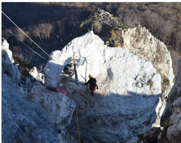
Figure 3. Drilling operation in view of blasting (right). Large impact caused by a rock block in the ditch. (Photos: Sage Ingénierie + S. Lambert)
