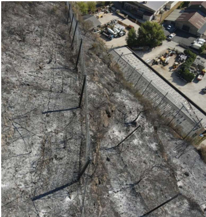
Figure 10 – View of the structures at Les Balmes; southern section (metal netting) upstream of the built-up areas. (Source: SDIS 38 – 9 August 2022)
