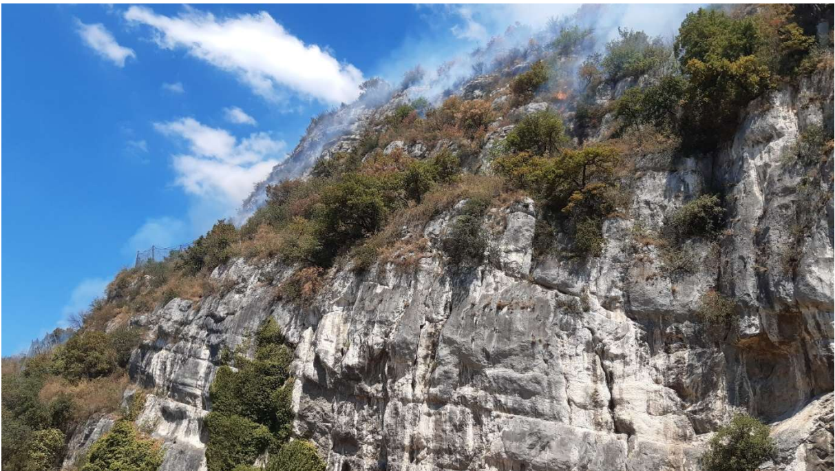
Figure 7 : limestone cliff above Impasse Lavoisier. (fire propagates in its upper part)
