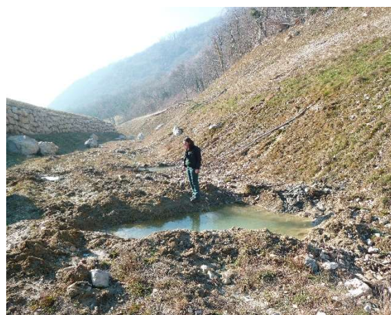
Figure 3. Drilling operation in view of blasting (right). Large impact caused by a rock block in the ditch. (Photos: Sage Ingénierie + S. Lambert)
