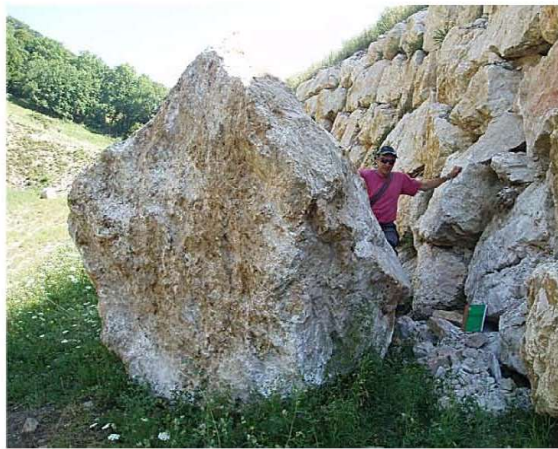
Figure 2. Rock block after interception by the embankment, after the natural event. Additional protection structure built in view of blasting (Photos: Sage Ingénierie)
