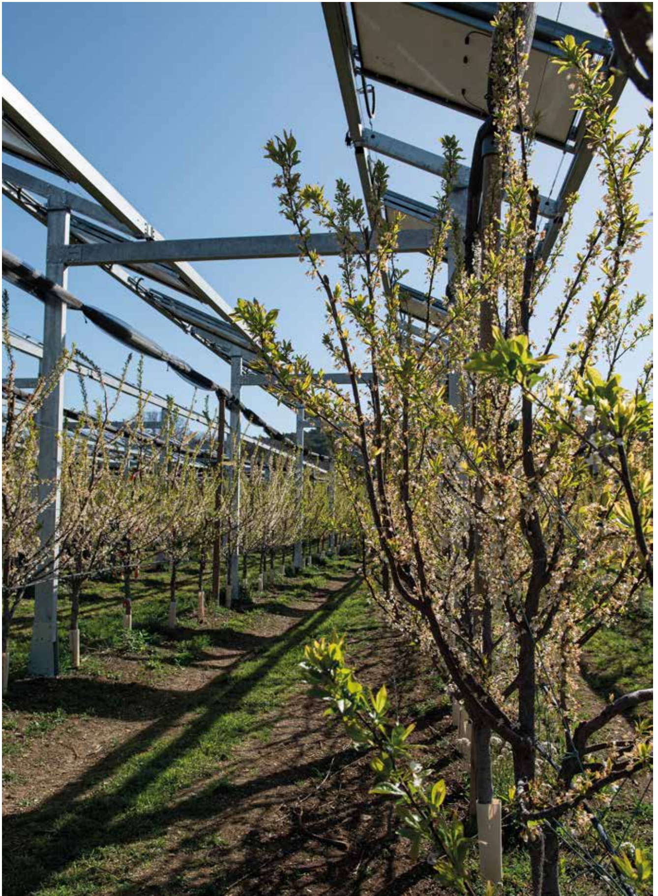
^ Solar panels casting shade on plum trees in a field near the town of Apt (Vaucluse); researchers are exploring how photovoltaic modules affect tree production. ©INRAE - B. Nicolas
